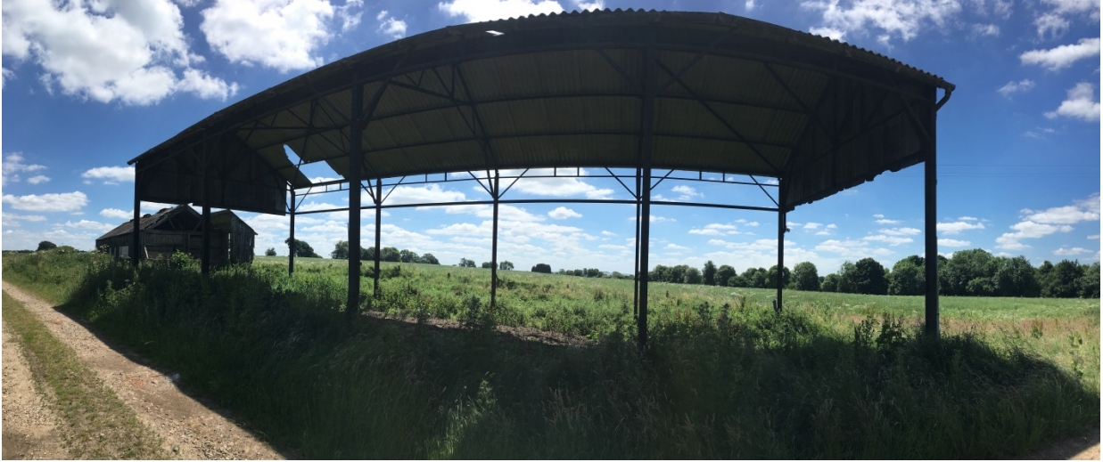
Photo 1: View of South (side) Elevation of Barn No. 2
