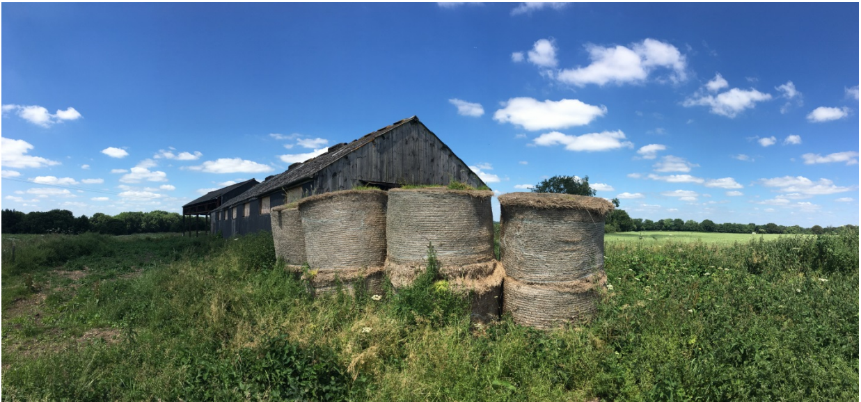
Photo 8: View of East (end) elevation of Barn No. 1
