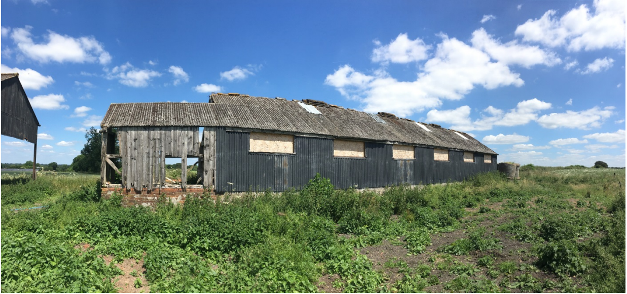
Photo 5: View of North (side) elevation of Barn No. 1
